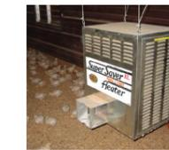
The inside mount model is a gas circulating heater ideal for a confinement environment.
